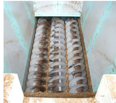
Mounting in discharge screw (wood-fired power plant)
